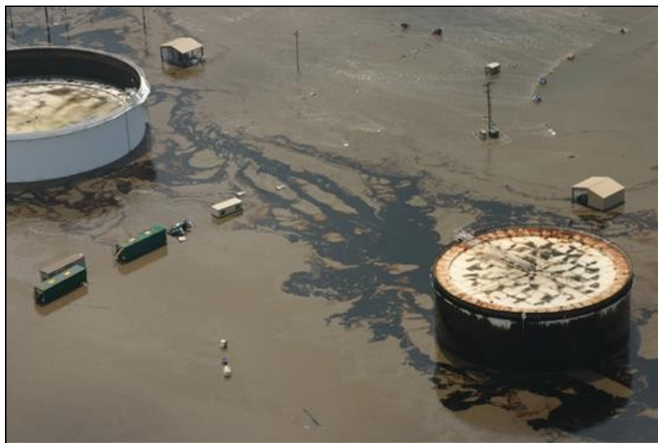
Image No. 13. – Oil spill formed after flood damage to storage tanks in Coffeyville, USA, in 2007. Source: Necci, Amos & Wood, Maureen & Krausmann, Elisabeth & Girgin, Serkan. (2020). Natech risk management Common Inspections Criteria.
