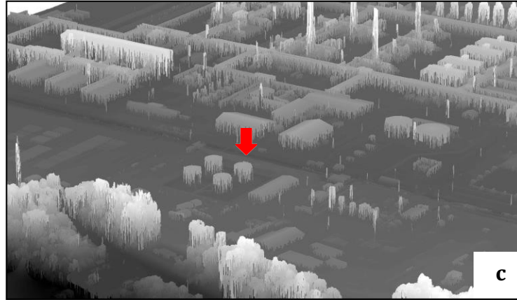
Image 16. a. Orthogonal photogrammetry of the gas plant. b. Digital surface modeling + Photogrammetry of the gas plant. c. Digital surface model of the gas plant. Note: In red arrow, affected storage tank. Source: SACS Consultores, 2022.
